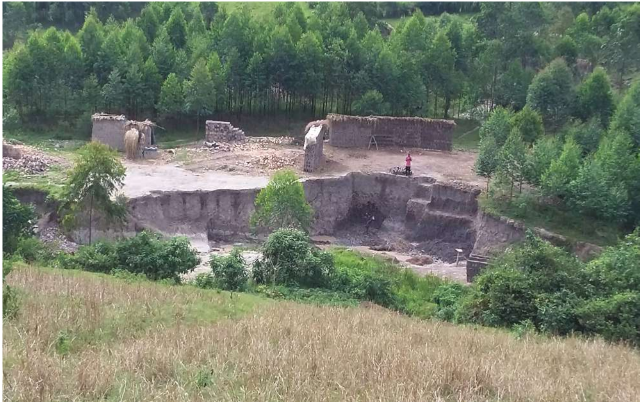
Plate 10: Brick making pits in Ikuniro village, Buhunga Sub-county
